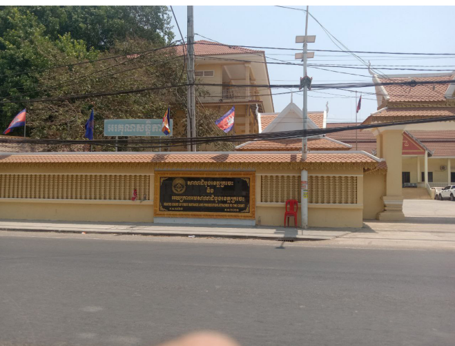
Kratie provincial court building on April 22, 2024. (Photo supplied)
